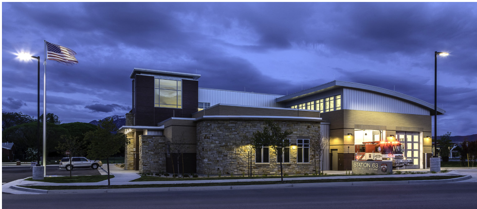
STATION 63 10451 SOUTH 1055 WEST
