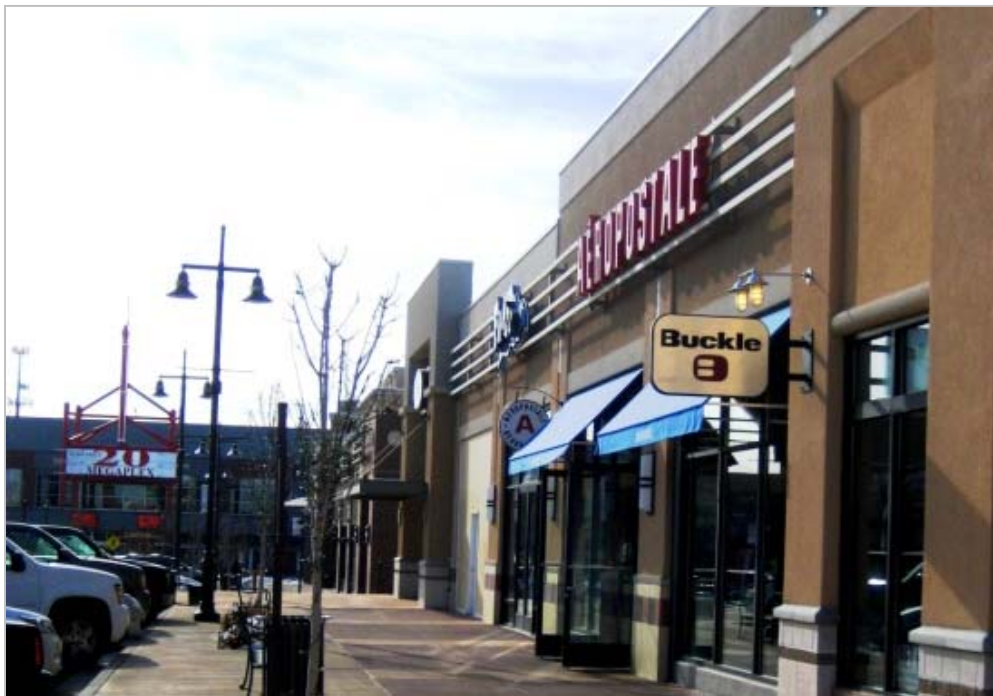
COMMERCIAL DEVELOPMENT AT THE DISTRICT
